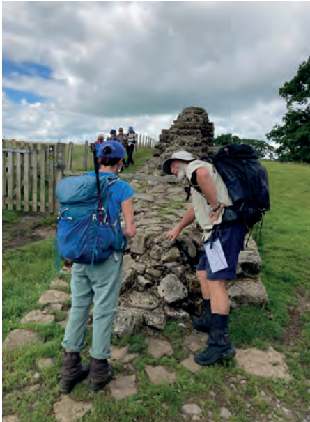
Discussion on wall construction
