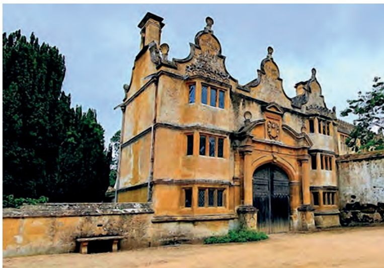
Gatehouse to Stanway Manor
